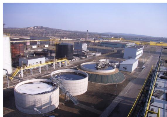
Fig. 2: Coke oven wastewater treatment plant with Mutag BioChip™ in Poland
