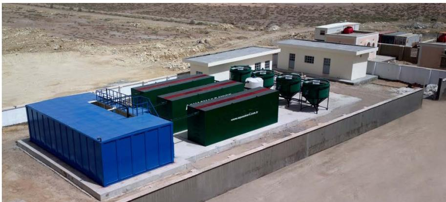
Fig 5: Containerized wastewater treatment plant operated with Mutag BioChip™, installed in Iraq in 2014
